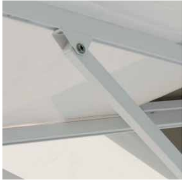
Scharniere einzeln verschraubt. Hinges are bolted separately.
